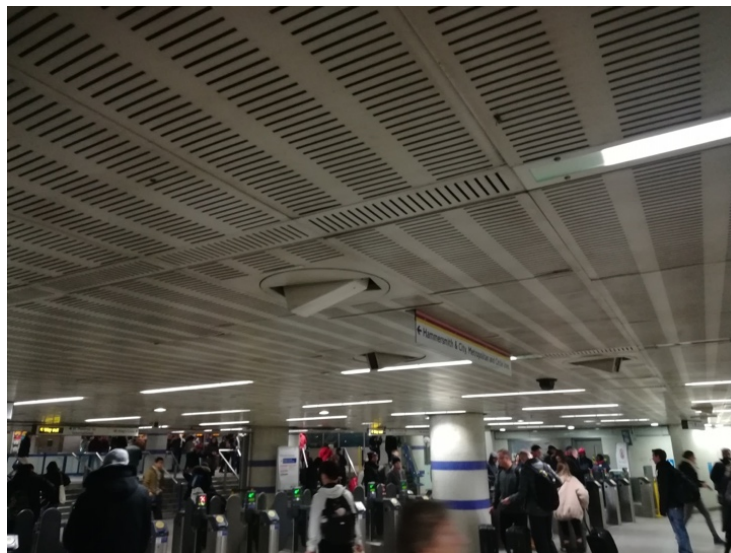
Fig 1. King's Cross St. Pancras Underground Station ticket hall. 6
