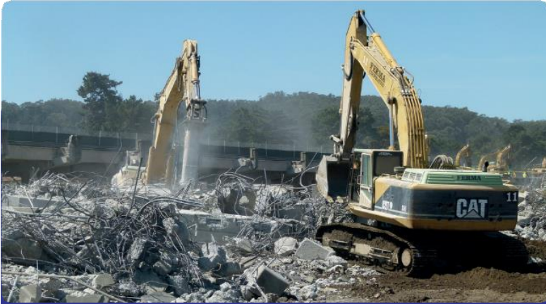
Site setup and demolition
