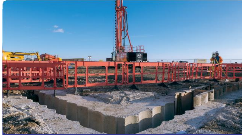
Basement excavation and piling
