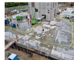
Well laid out site with demarcated walkways.
