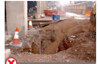
open excavation next to roadway
